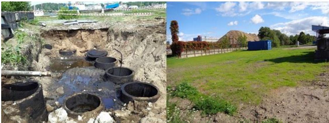
Sarkandaugava’s Site before and after performed remediation works
